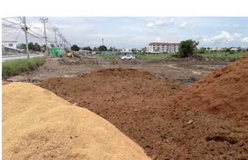
3rd Month Highly-fertile engineered soil imported into the site to prevent compaction and allow for porosity of the designed
